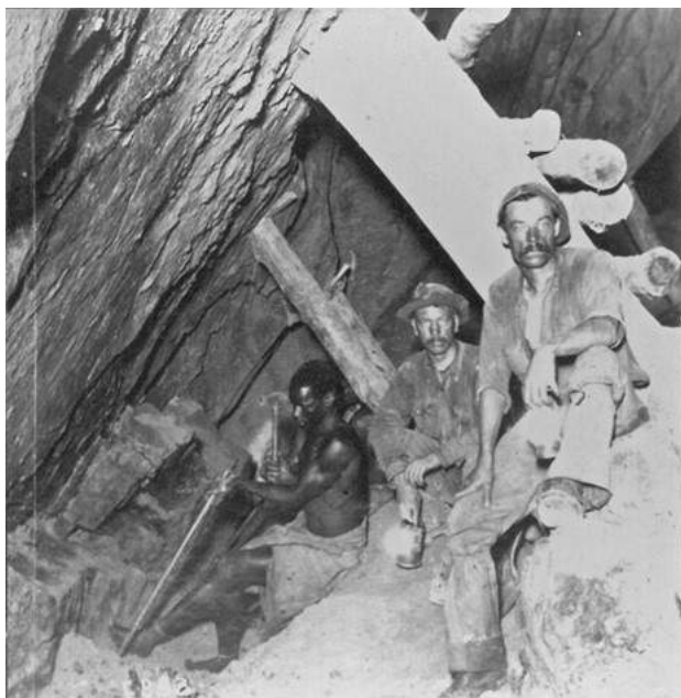
Very steeply dipping strata, and steep-angled timber supports. Virtually all the photos show European miners with some or other form of soft hat or cap, and with ubiquitous droopy moustaches. Here both of them are holding lit carbide lamps. Note the barefooted African worker. Crown Mines C832.
