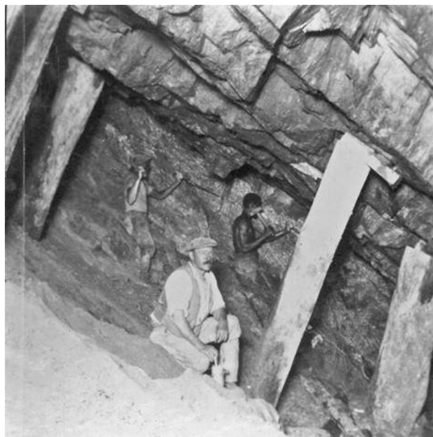
This photo shows one of the pair of stereo photos. Two labourers are chipping away at the reef behind the seated miner. Note the dip on the rocks, the timber roof supports, and the carbide lamp in the miner's right hand. Crown Mines C858.
