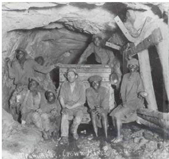
Hand written label reads: "Tramming, Crown Mines C240". Again, note the barefoot labourers and the low, narrow workway. The labourer on the right appears to be holding a candle, while the one front-left has a carbide lamp.
