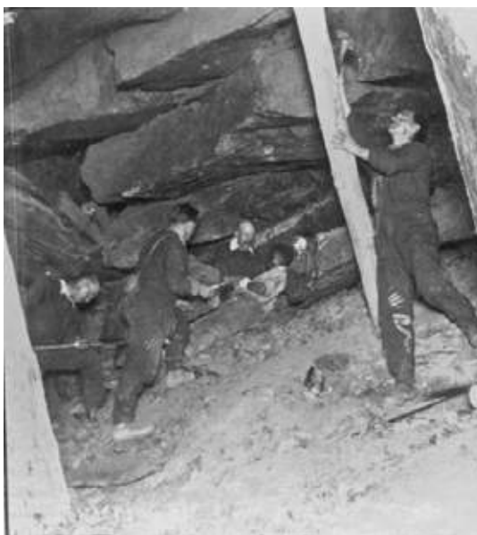
Sampling the reef at Crown Mines. Sections have been marked off using chalk to delineate the sample intervals. The miner (geologist?) can be seen hammering with a steel chisel while the labourer sits holding a container to catch the fragments. A second miner sits and records the sampling.
