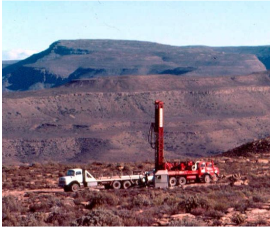
Schramm percussion drilling rig in action on the escarpment.
